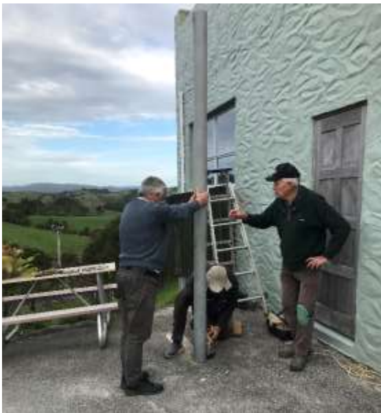
Outer skin is cut but base pole does not move
