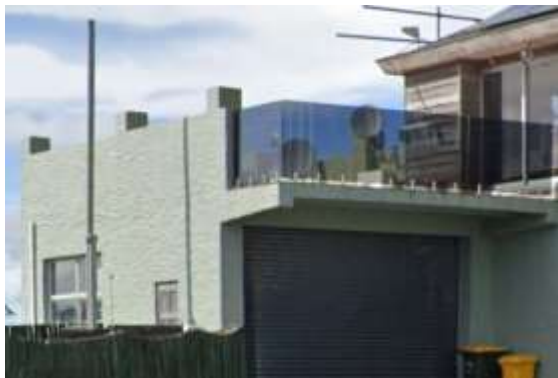
Tilt-over mast at Clevedon house
